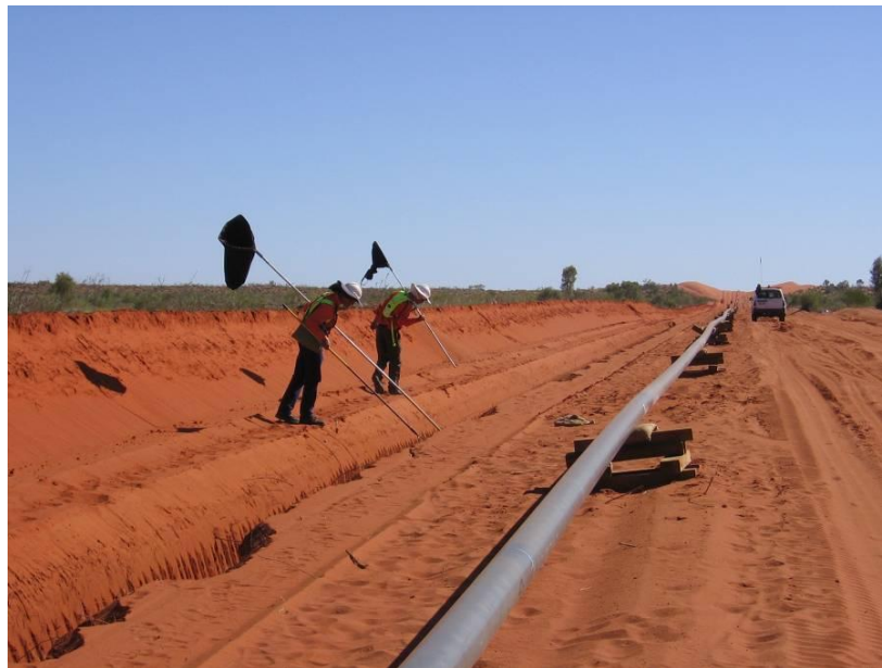
Plate 2: Pair of Fauna Officers inspecting Open Trench
